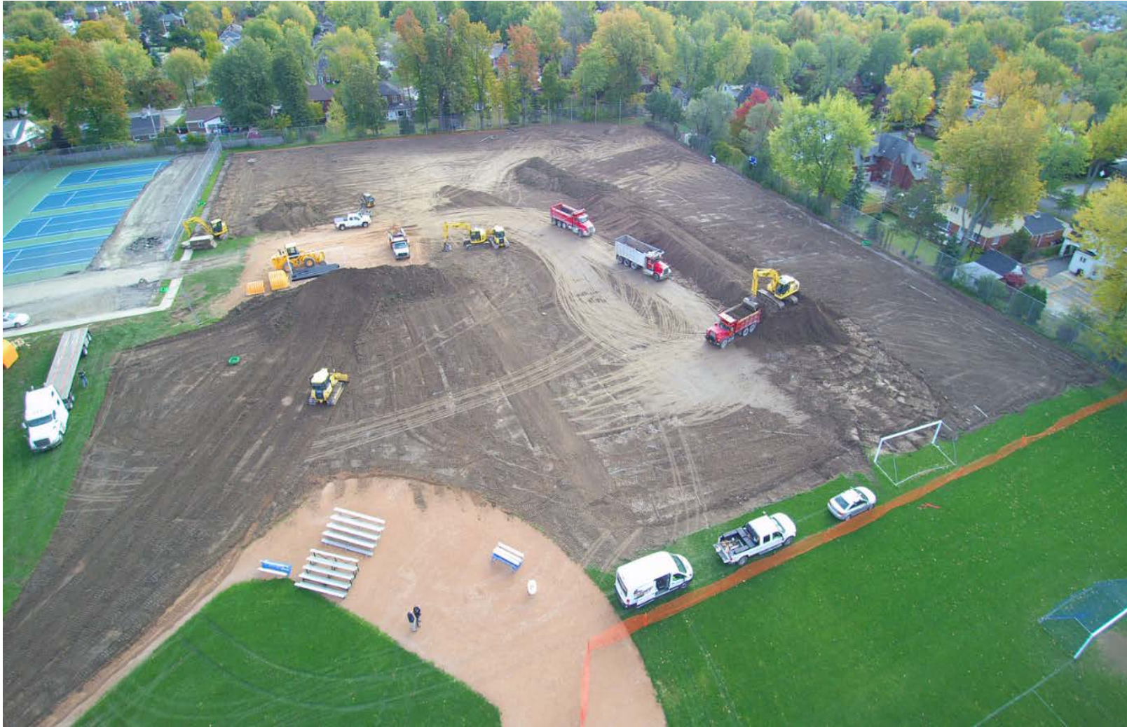
Site Preparation at Kenmore West High School Field
